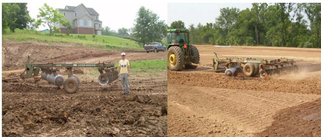
Fig. 1. The picture shows (a) the disking equipment used to create microtopography and (b) how the disking was conducted, all during the construction of Loudoun County mitigation bank wetland.
